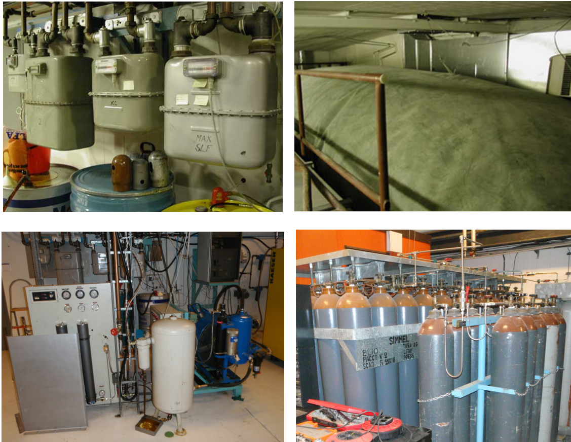
Figure D.4: Upper left: The gas flow meters measuring return gas. Upper right: The gas bag. Lower left: Gas compressor. Lower right: The storage of incoming gas.
